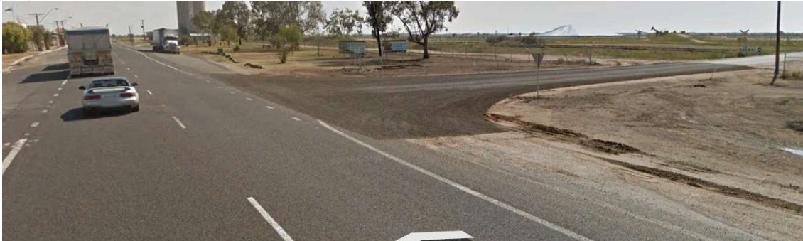
Figure 8: Sight distance along the Newell Highway intersection exceeds the minimum requirements
